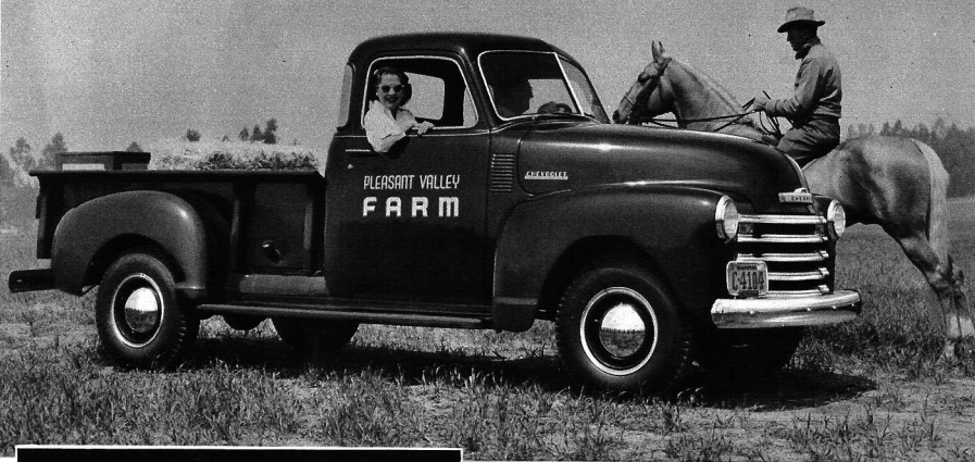
MODEL 3604 "DE LUXE" PICK-UP 125 3/4-INCH WHEELBASE, MAXIMUM G.V.W. 5800 LB.
